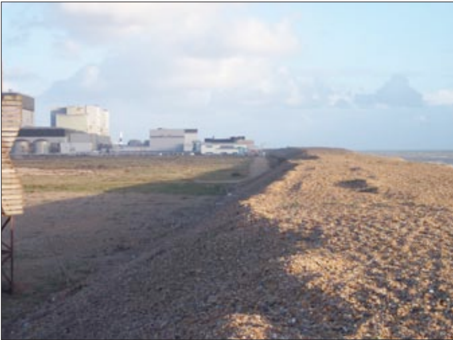
Photo 1. Profiling of the gravel ridge at the nose of the foreland attempts to safeguard the power stations. However, with increasing storm surge heights, re-profiling may result in over-steepening. This increases the susceptibility to barrier breakdown and breaching, which would result in widespread flooding of the area.
