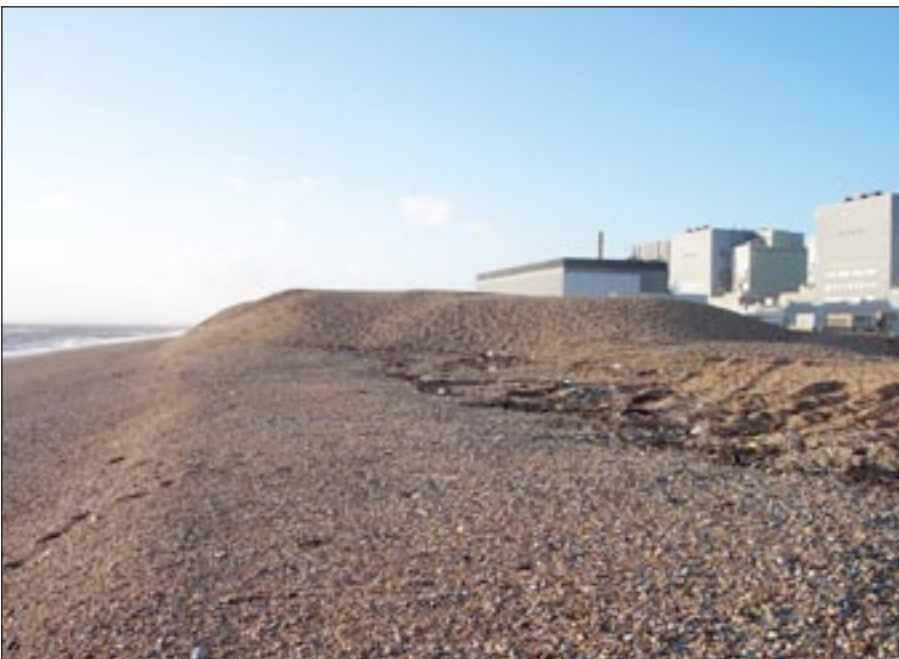
Photo 2. 60,000m 3 per year of shingle is recycled from the east-facing to the south-facing side to maintain the fixed plan of the shoreline.
