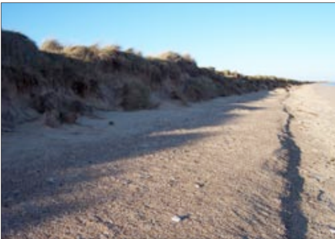
Photos 10 and 11. Climate change is likely to have the greatest impact at the northern end of the system at Sizewell, resulting in possible breaching where dunes hinge on the cliff line and flooding of low-parts of Minsmere.
