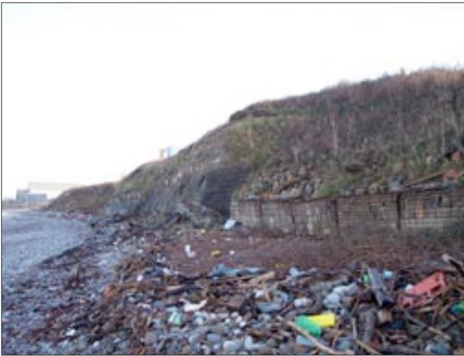
Photo 5. Additional cobble gabions protecting sections of the cliff to the west of the station.
